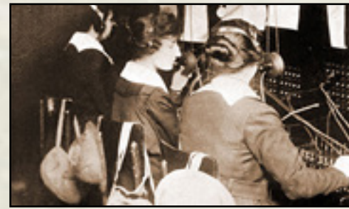
ON DUTY: 'Hello Girls' operating a switchboard. Note the ever present air raid kits within easy reach.
